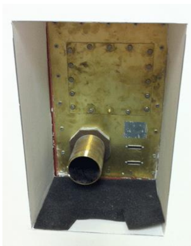
Figure 13: Typical penetration panel with waveguide tube and 15 pin d-type cutouts (bottom right of the image)
